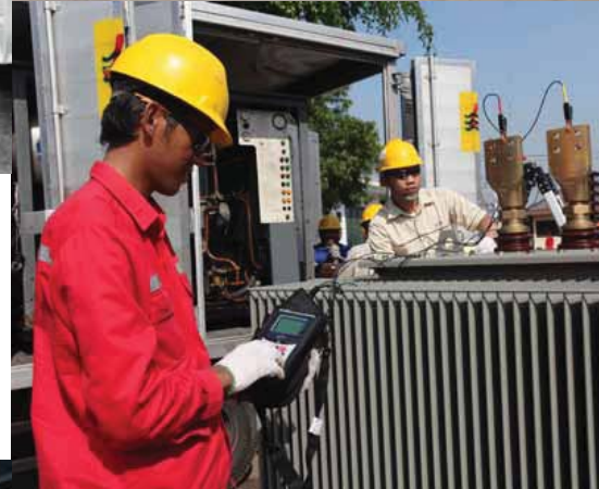
◀ Transformer testing and commissioning
