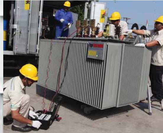
◀ Transformer oil treatment
